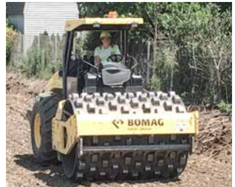
COMPACTING soil on the I-75 reconstruction project in Findlay for Shelly & Sands is Nicole Fastzkie.
