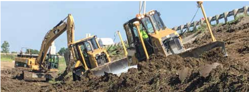
STRIPPING slopes on S.R. 15/68 on the I-75 reconstruction project in Findlay for Beaver Excavating is Jason Kramer in the hoe, apprentice Layla Dia in the left dozer and Ken Eckleberry in the right dozer.
