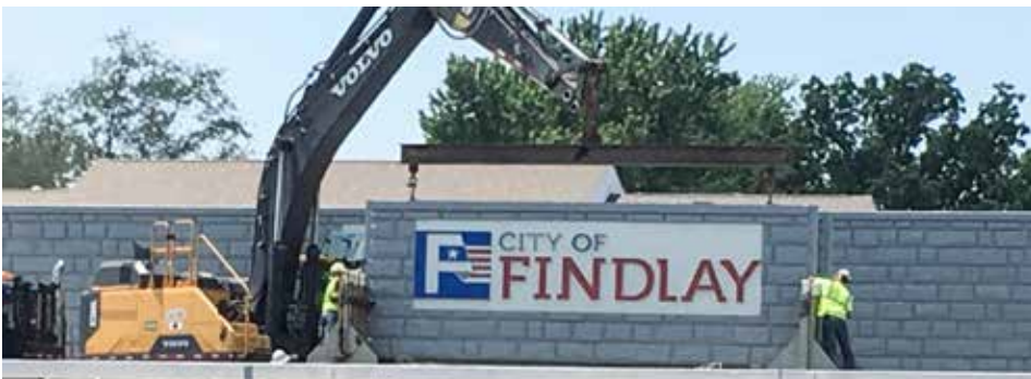
INSTALLING a noise wall in Findlay on the I-75 third lane project for Shelly & Sands is Jeff Stechsulte.
