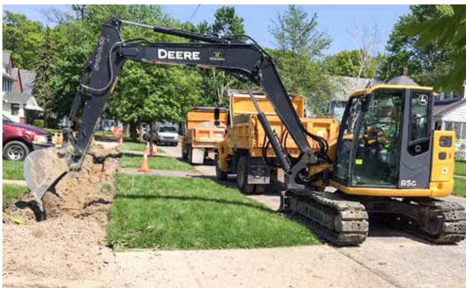
RUNNING an excavator backfilling a gas line ditch for Miller Pipeline on Princeton Avenue in Elyria is Paul Bores.
