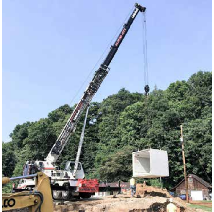
OPERATING the crane for Capital City Crane in Lawrence County for Axis Civil is Jim Spohn, while Steven Pack is signaling sitting a box culvert.
