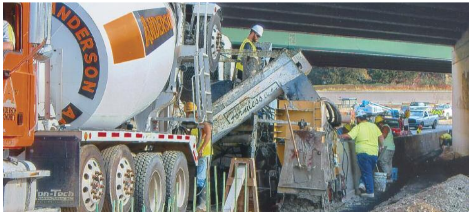
COMPLETE GENERAL slipping wall on I-270/U.S. Rt. 33 reconstruction in Dublin.
