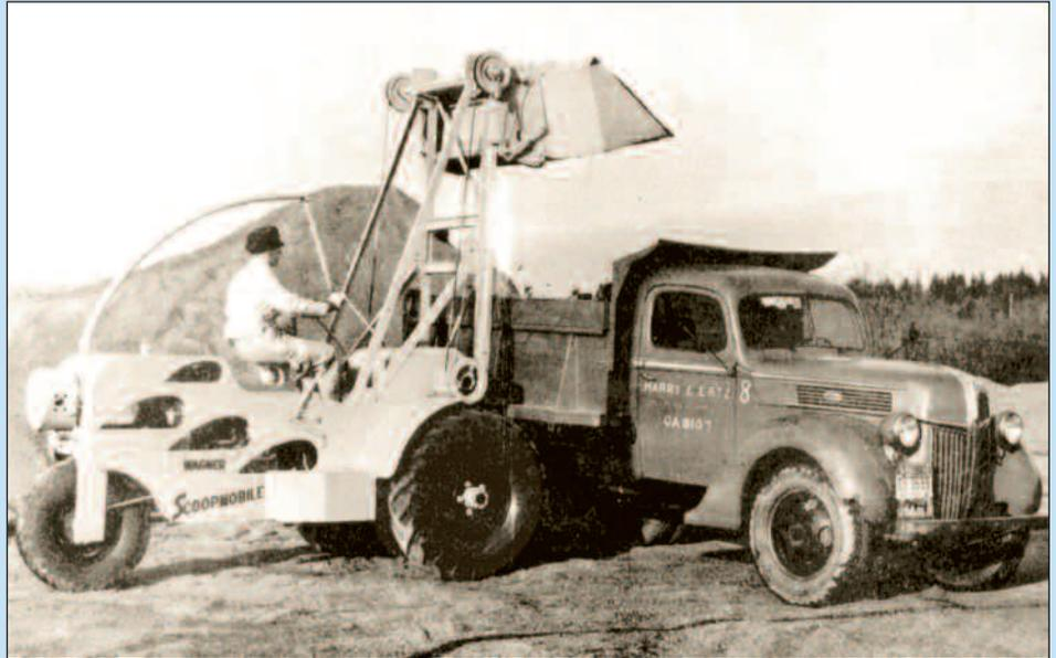
**THREE-WHEEL LeTourneau loader. The first purpose-built wheel loader was invented in 1939, a new piece of equipment for the newly created Local 18. For years the loaders were cable-operated and bucket capacity was a cubic yard or less. The bucket would be tripped for dumping then had to be reset for another load.**
